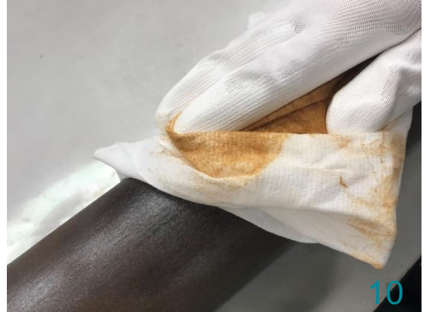
Continue until the surface is clean and all contaminations have been removed
