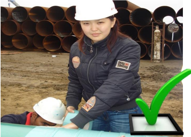
Apply Wrappingband without tension.
