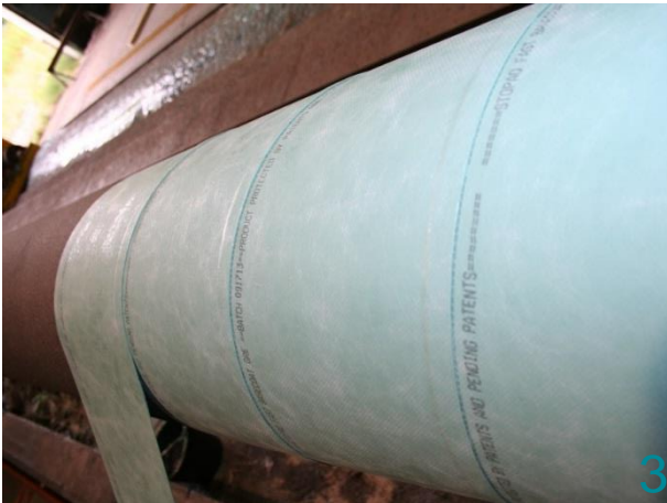
3 The overlap can be adjusted by changing the travel speed of the FAST Basecoat Wrapping Device. New rolls shall be installed with a minimum circumferential overlap of 50mm.
