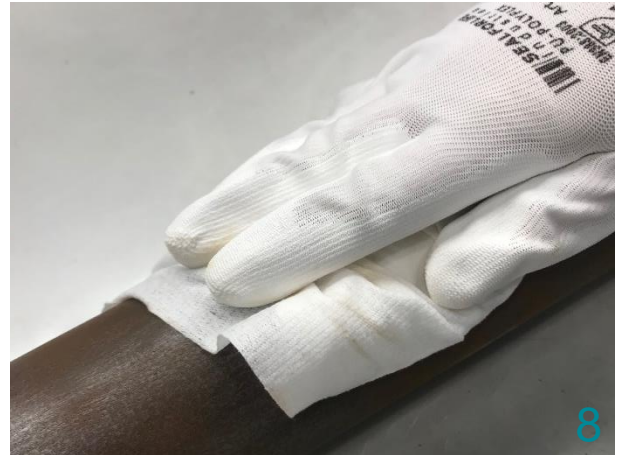
After folding the SFL Cleaning Wipe the surface can be cleaned. Firmly rub the entire surface with the Wipe
