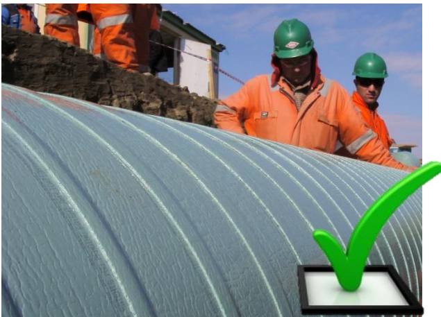
Minimum side by side overlap shall be 10mm. Respect the printed indication line on the Wrappingband, present on the Wrappingband wider than 50mm.
