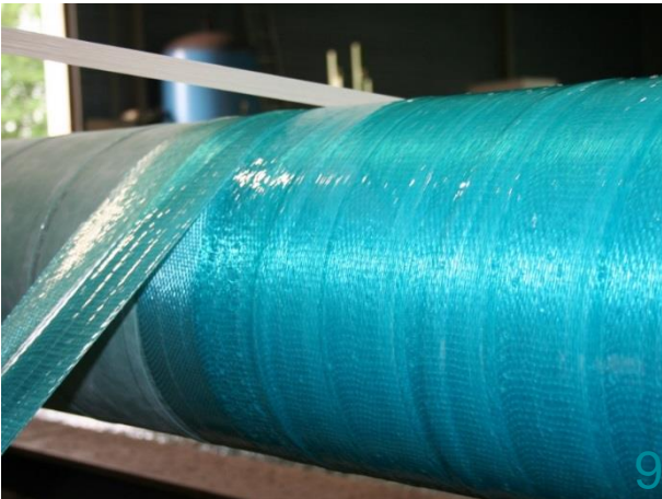
STOPAQ FAST GRE Surface Veil is the outer layer of the STOPAQ FAST GRE System.
