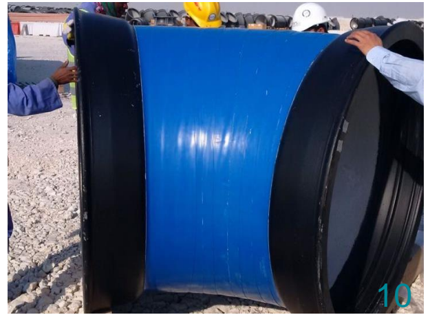
Apply the last part of the SynergyQ® Ductile Iron Wrapping Tape without tension and firmly press the material in the pores of the substrate
