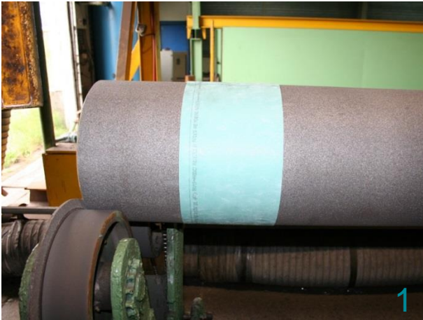
1 After surface preparation, straight wraps of Stopaq FAST Basecoat GRE shall be applied at both sides of the pipe, minimum 200mm from the pipe end.
