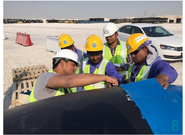
Consecutive overlap when a new roll is used minimum 300mm
