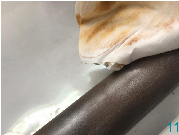
Surface cleaned with SFL Cleaning Wipe.
